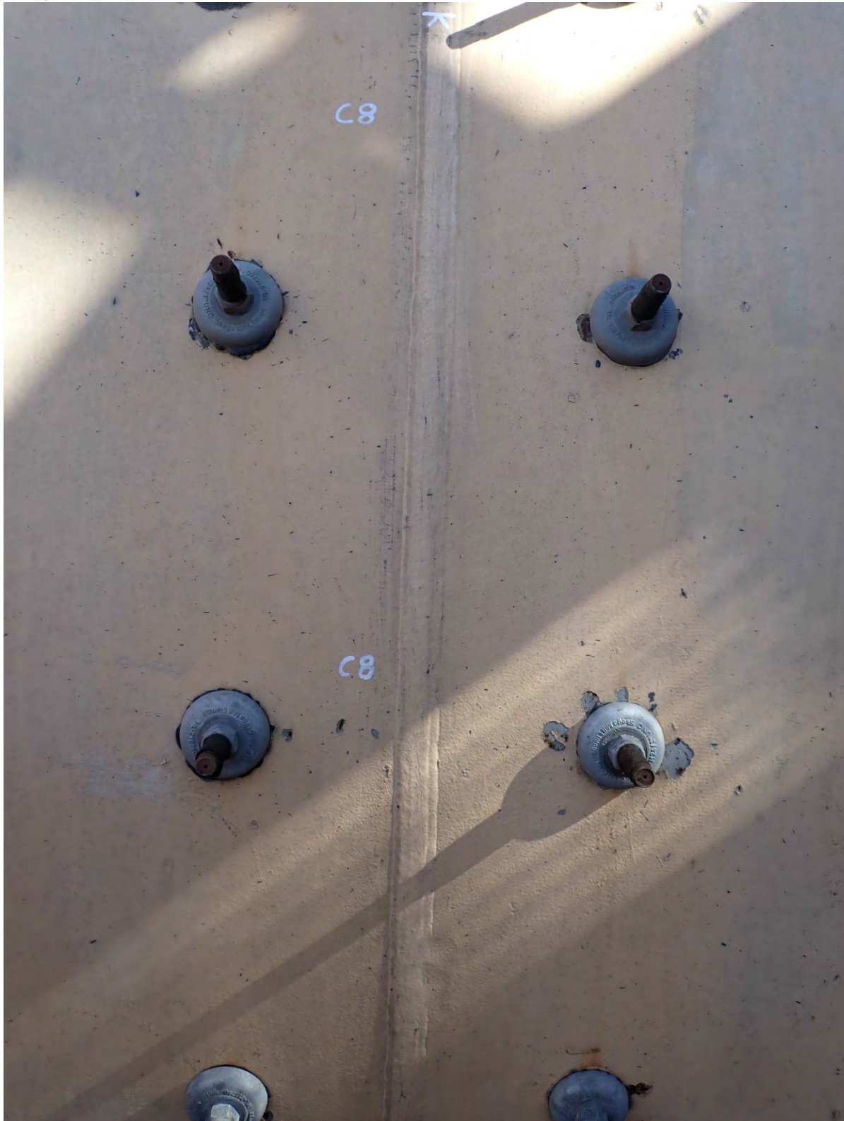
Circumferential weld at inspection run 8
