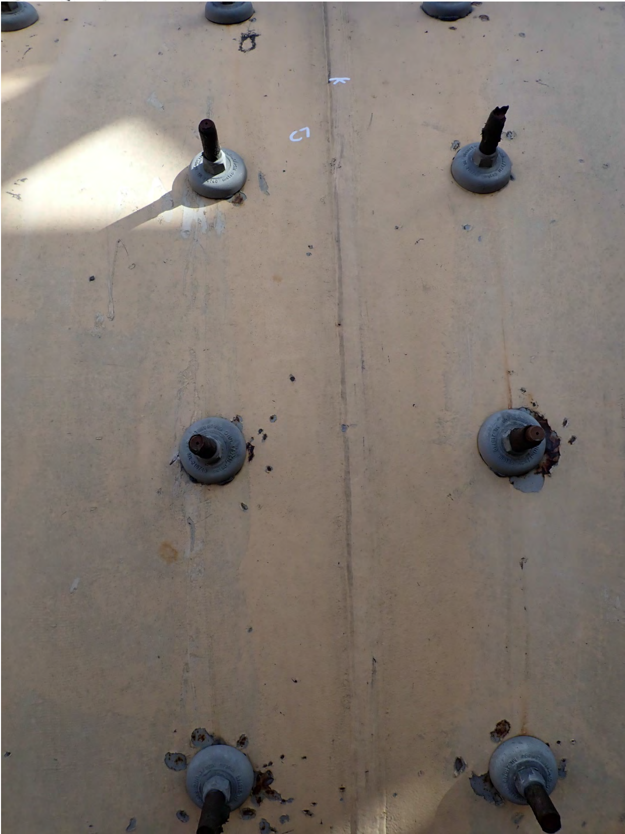
Circumferential weld inspection run 7
