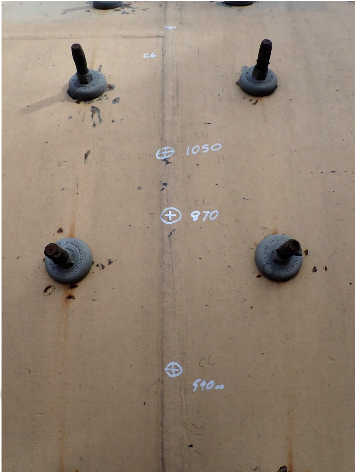
Circumferential weld run 6
