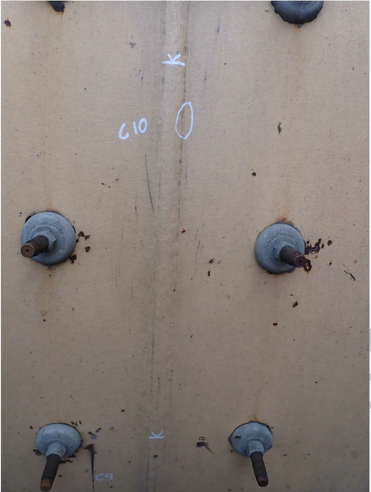
Weld inspection run 10
