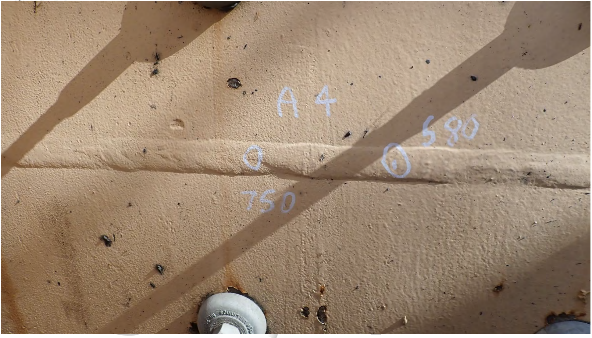
Axial weld discharge end 2 nd run
