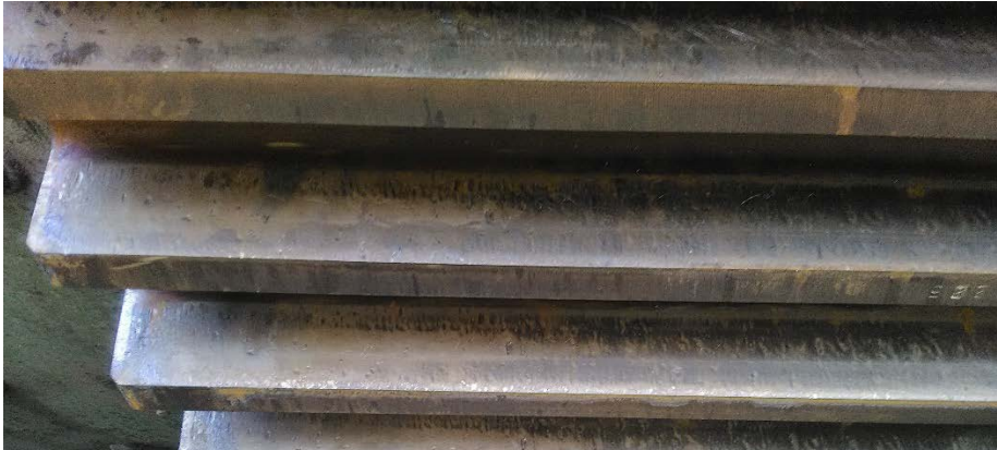
Fig 1 Gear tooth cleaned before remedial work commenced (Drive end).
