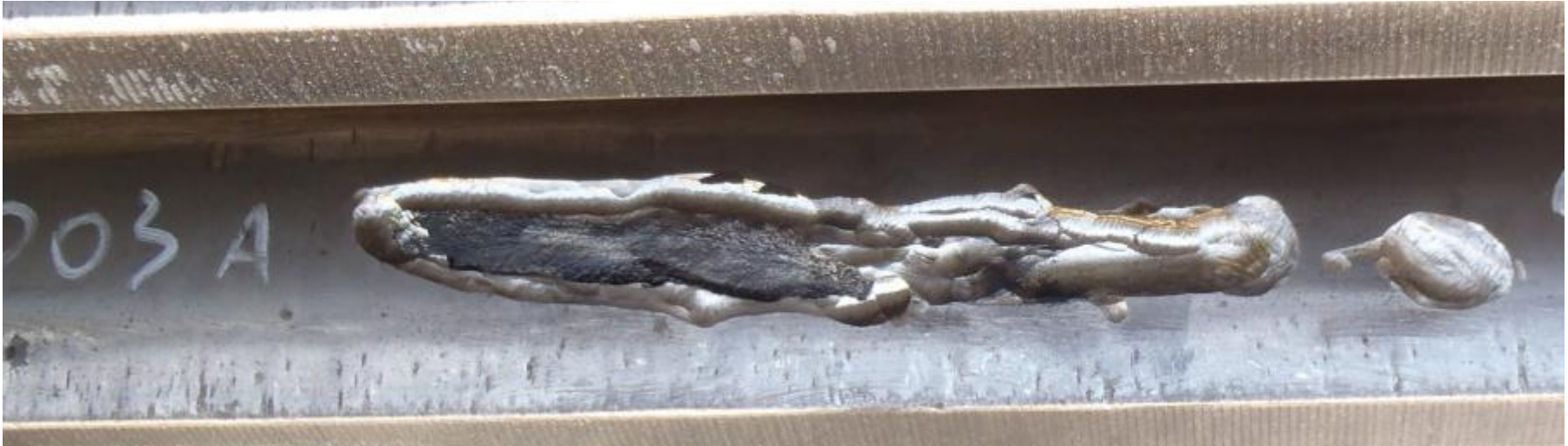
Fig 9 first stage of excavation – a chunk had cracked under the surface (dark grey area)
