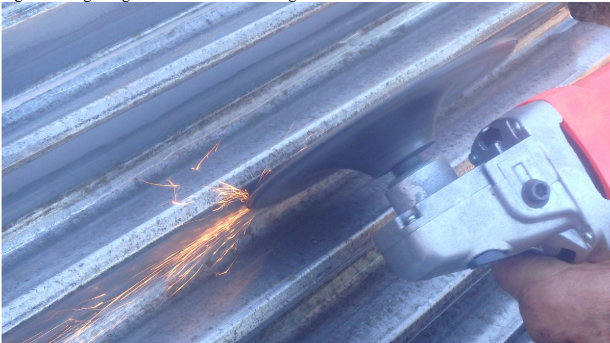
Fig 4 Sanding using a flexible backed sanding disc
